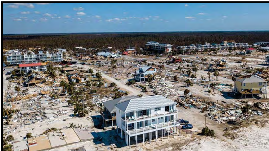
ICF home surviving a 250mph hurricane on Mexico Beach Florida
